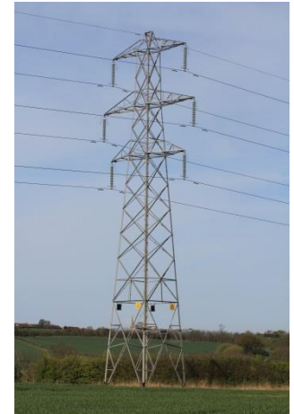
132kV DC lattice
